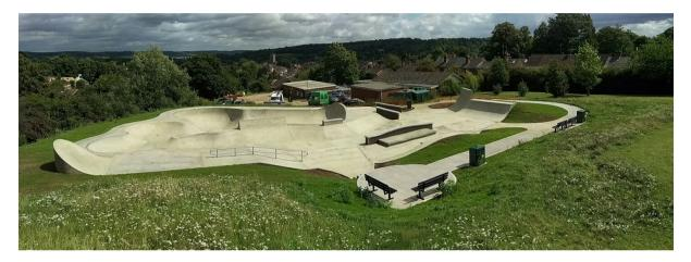
The concrete is uncoloured and once cured presents a light grey appearance. There are elements of bright steel work within the park which are there to protect edging and avoid chipping when the park is in use. You can see where by inspecting the attached visuals.
